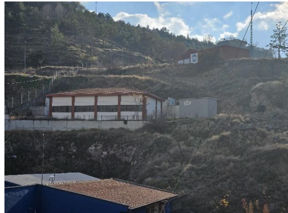
Existing Water Tank
