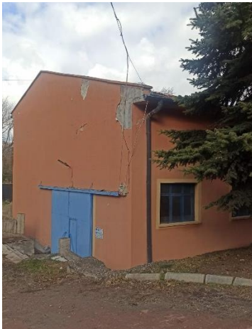
Water Pump Building
